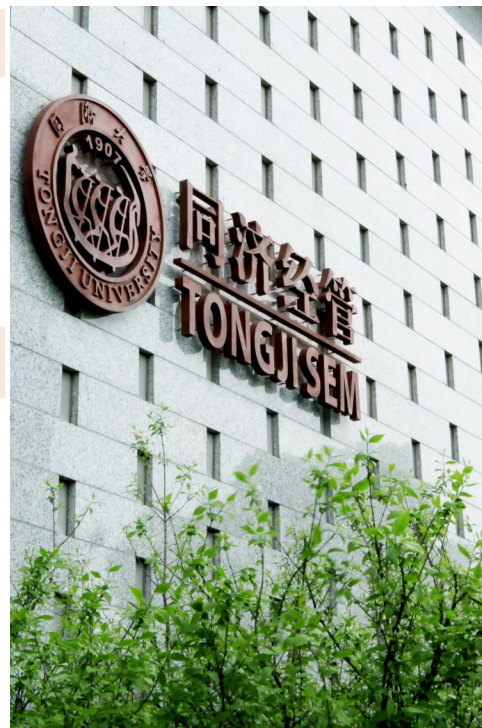
Tongji Building A
